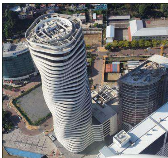
Figura 58. Vista superior Torre The Point, Guayaquil.
