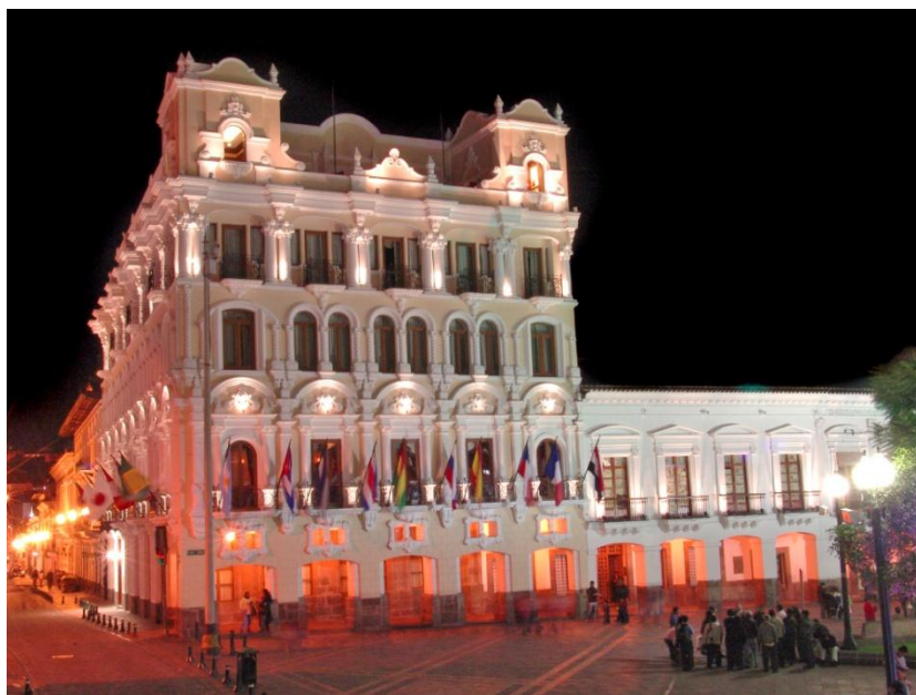
FOTO 2.62 FACHADA PRINCIPAL HOTEL PLAZA GRANDE
