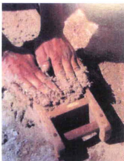
DC17 Relleno moldes
