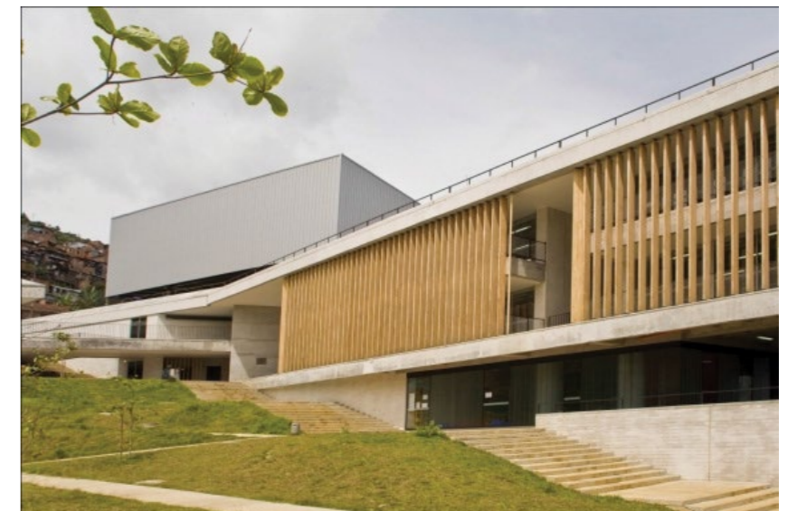
Figura 49. Colegio Antonio Derka, Santo Domingo, Colombia. Tomado de (Newbogota in Arquitectura, s.f).
