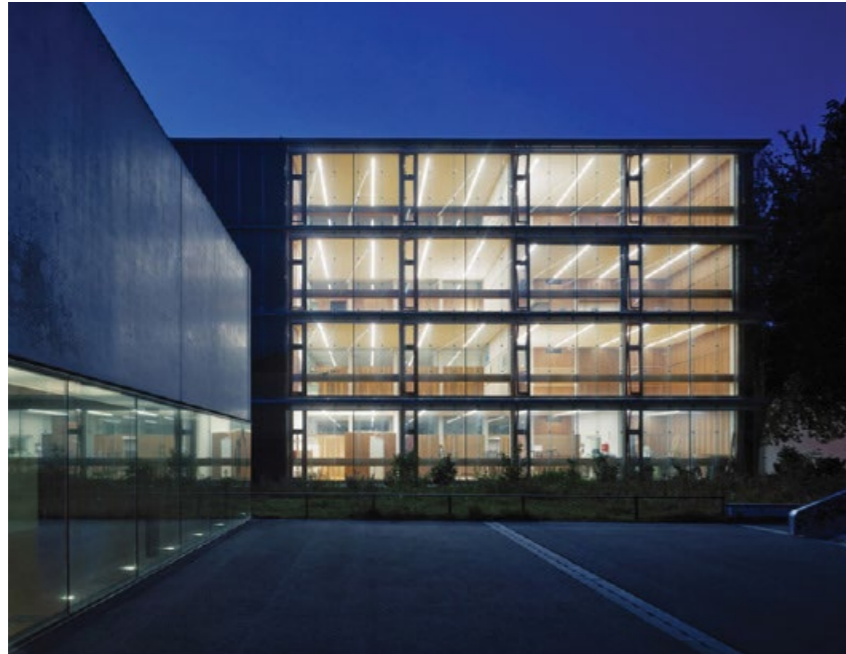
Figura 50. Colegio Mader, Austria. Tomado de (Baumschlager, s.f).
