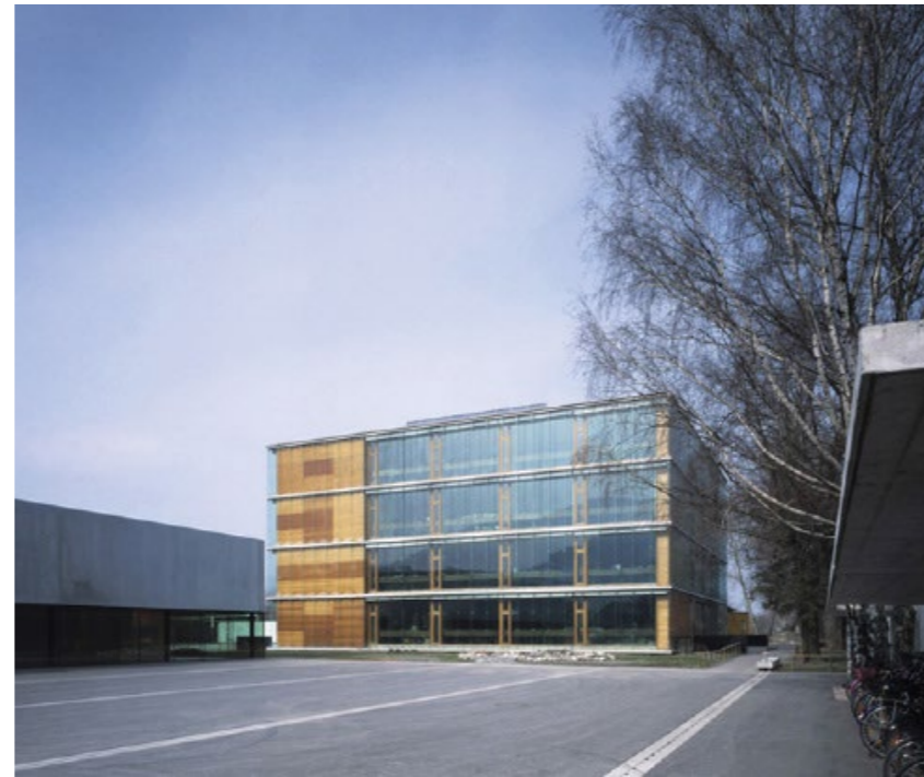
Figura 54. Colegio Mader, Austria. Tomado de (Baumschlager, s.f).
