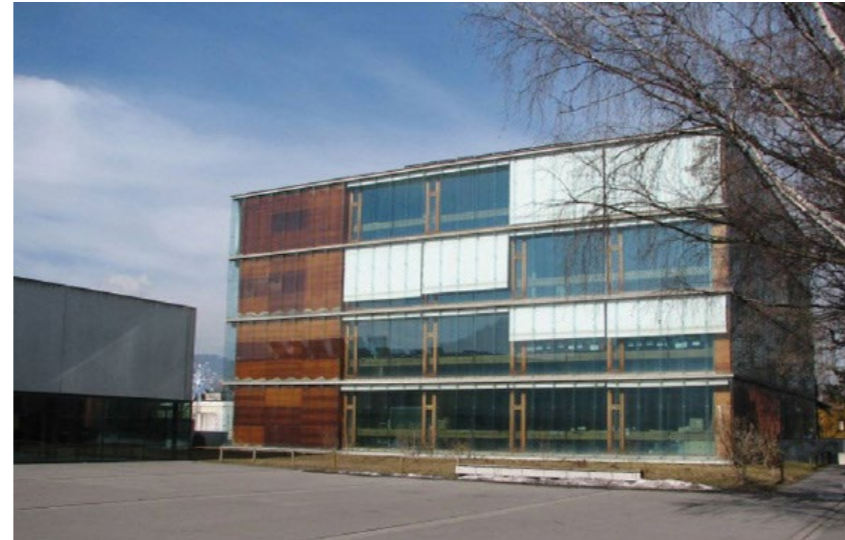
Figura 46. Colegio Mader, Austria. Tomado de (Baumschlager, s.f).
