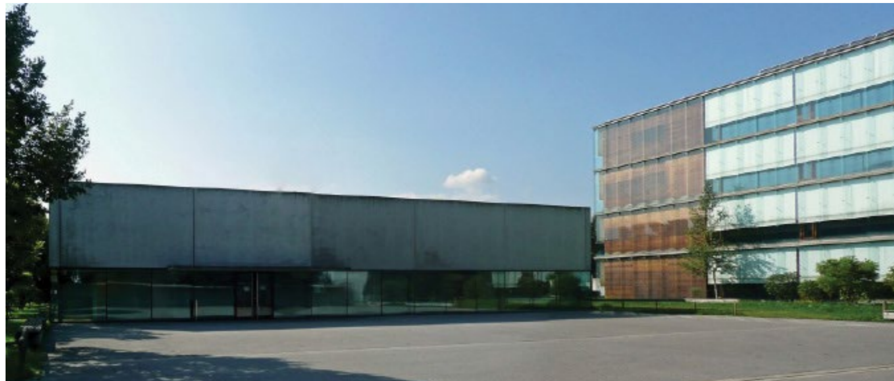
Figura 53. Colegio Mader, Austria. Tomado de (Baumschlager, s.f).
