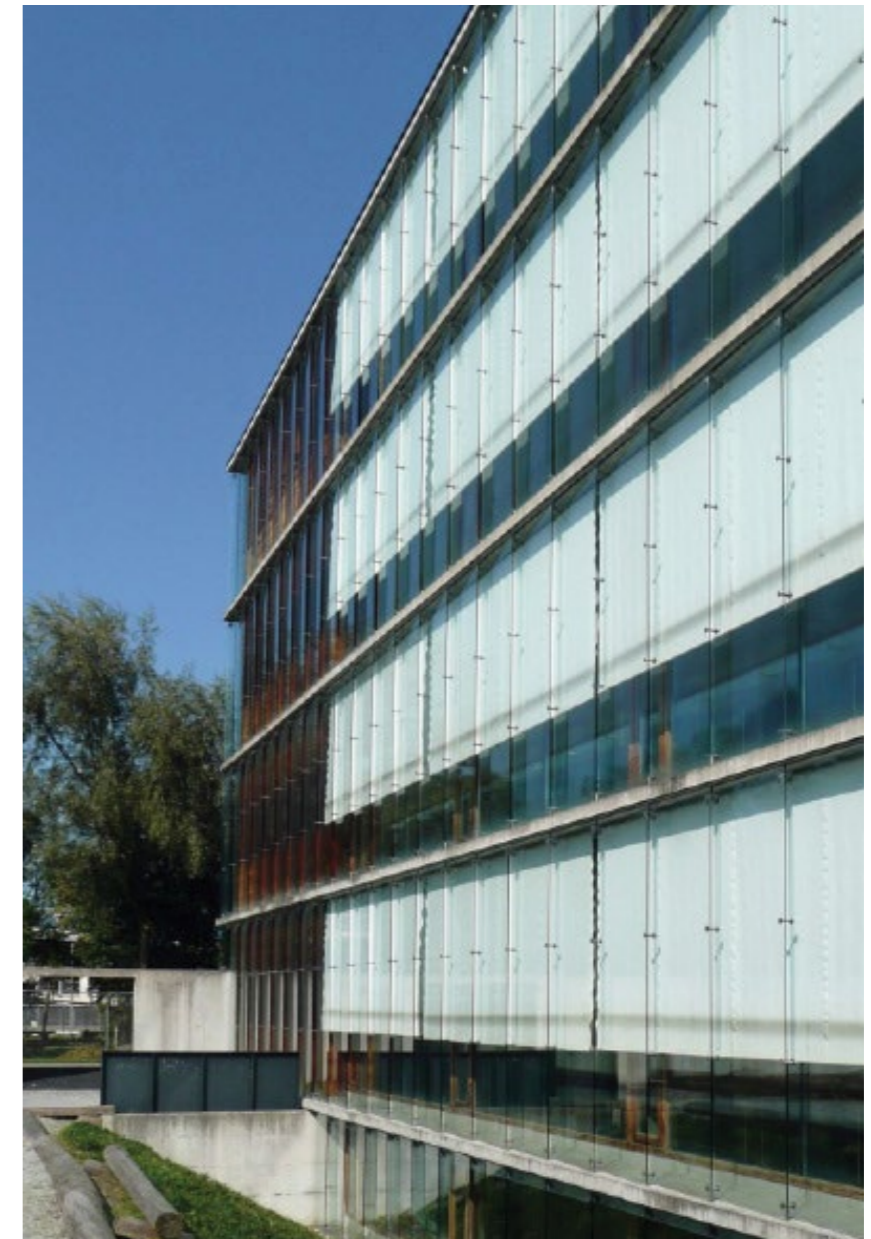
Figura 52. Colegio Mader, Austria. Tomado de (Baumschlager, s.f).
