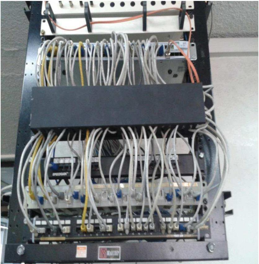
A close-up photograph of a network patch panel. The panel is filled with many white and blue Ethernet cables plugged into the ports. A black horizontal bar is mounted across the top of the panel. The panel is mounted on a black metal rack. The cables are organized in a somewhat chaotic manner, with many loops and crossings.                                                                               |
