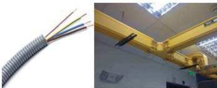
Figura 78 Tubo corrugado y fiber runner
