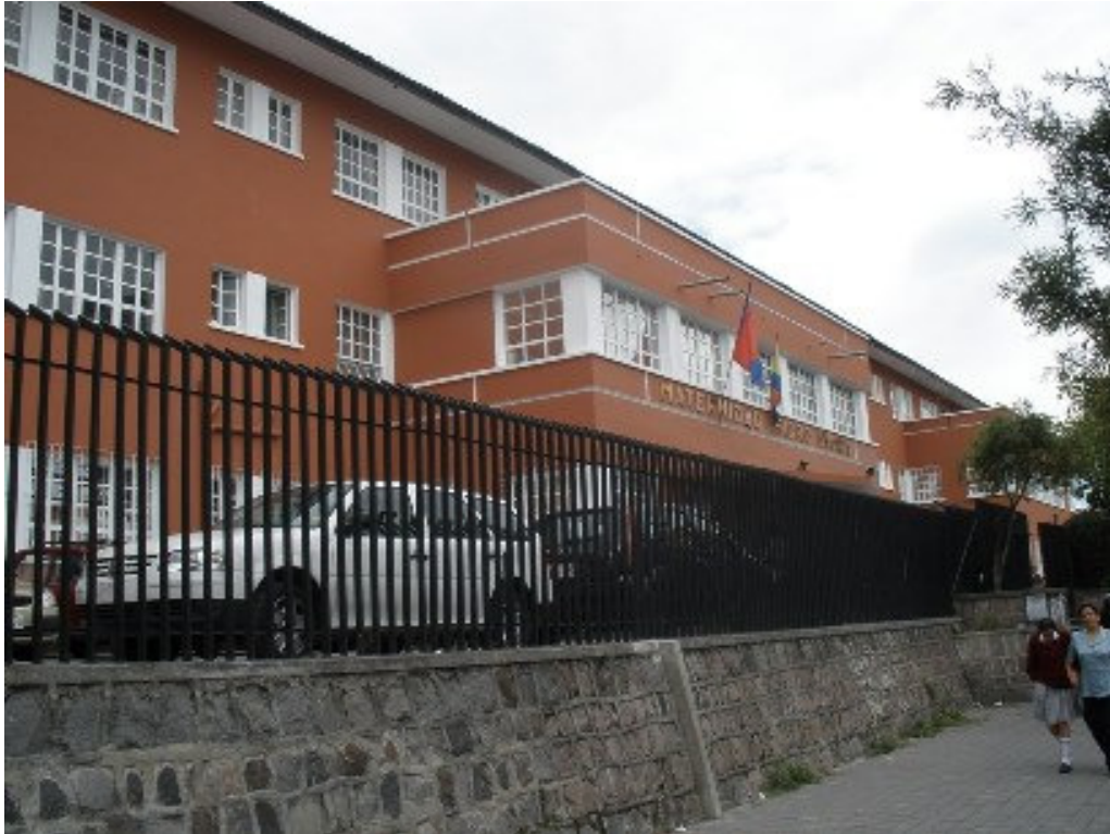
Hospital Gineco Obstetra Isidro Ayora
