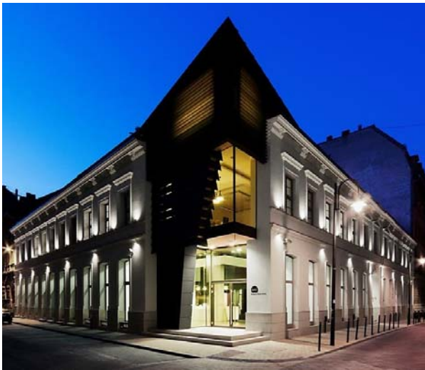
Figura 15. Budapest Music Center. Fachada exterior.
