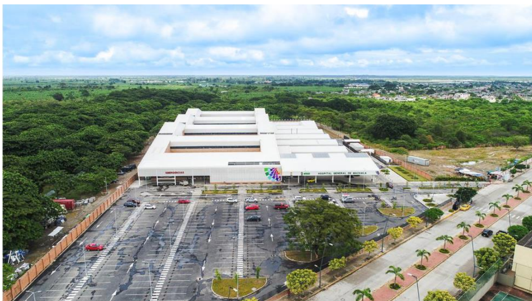
Figura 1. Hospital General Machala.
