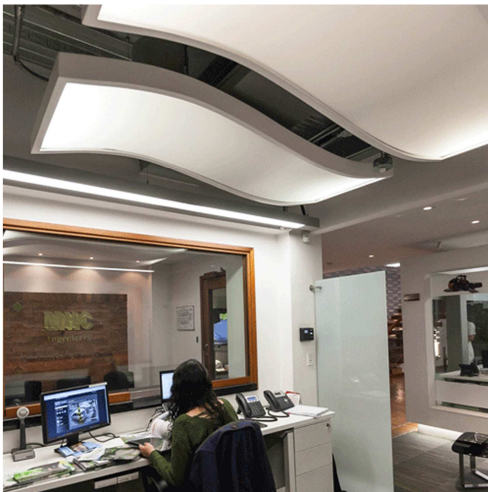
Figura 6. Cielo raso tensoflex tomada de (High lights, 2018)
