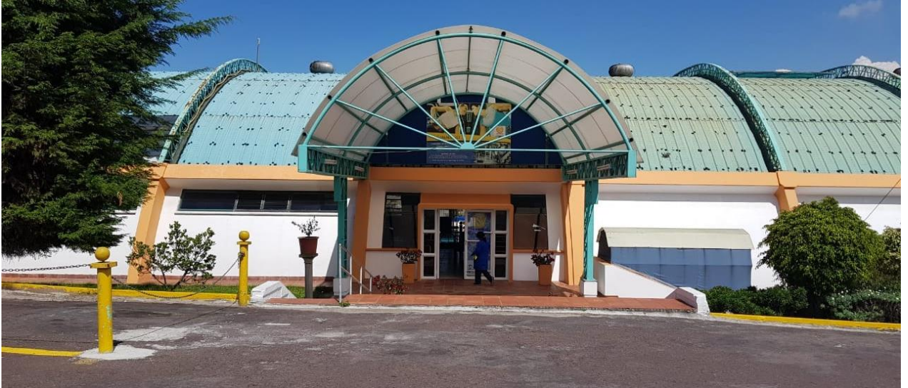
Figura 1 Fachada Frontal Club recreativo Rancho San Vicente
